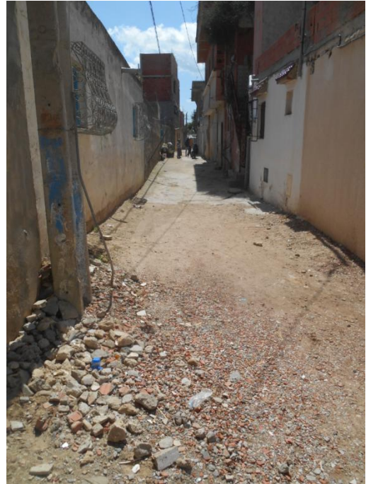
Voie 5 (36°42'3.04"N/ 10°31'27.66"E)
